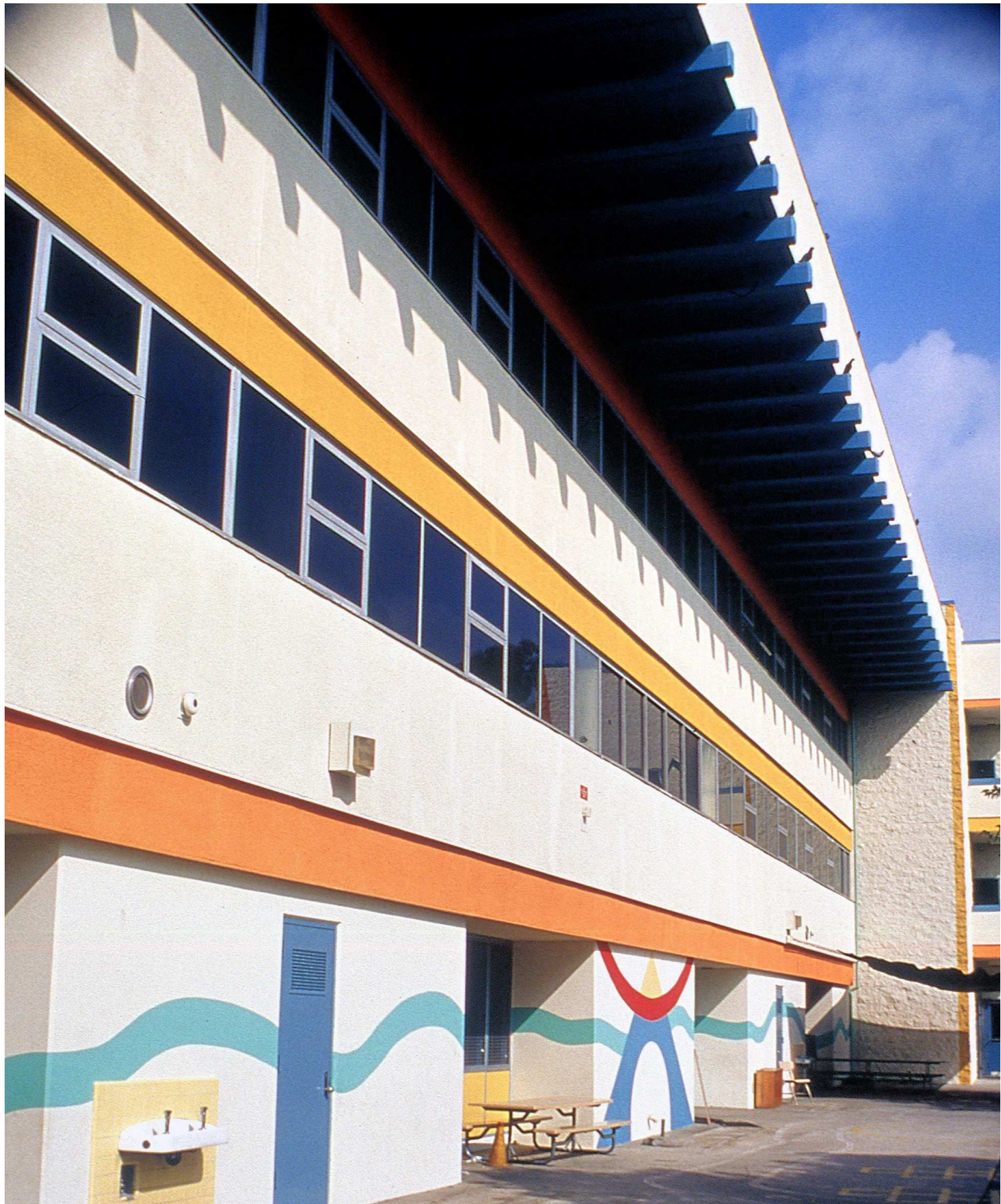
10TH STREET ELEMENTARY SCHOOL- DETAIL
